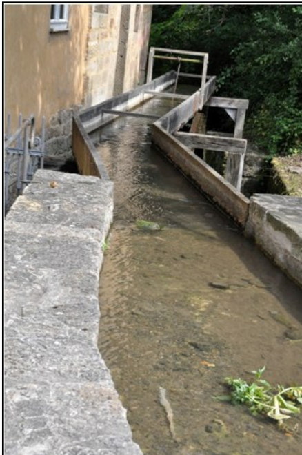
The Reß Mill: Left, the long water trough; center, the waterwheel with water flap; right, trough overflow
