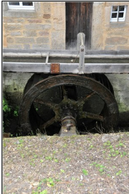
The Reß Mill: Left, the long water trough; center, the waterwheel with water flap; right, trough overflow
